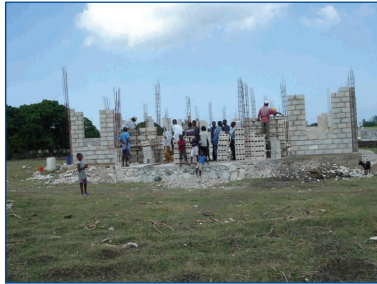
Present construction of Santo Church
