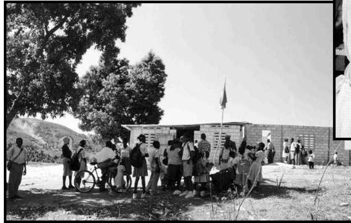
A rural school under construction.
