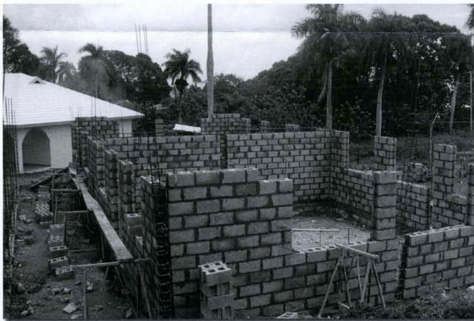
The construction of the Library and Computer Lab.
