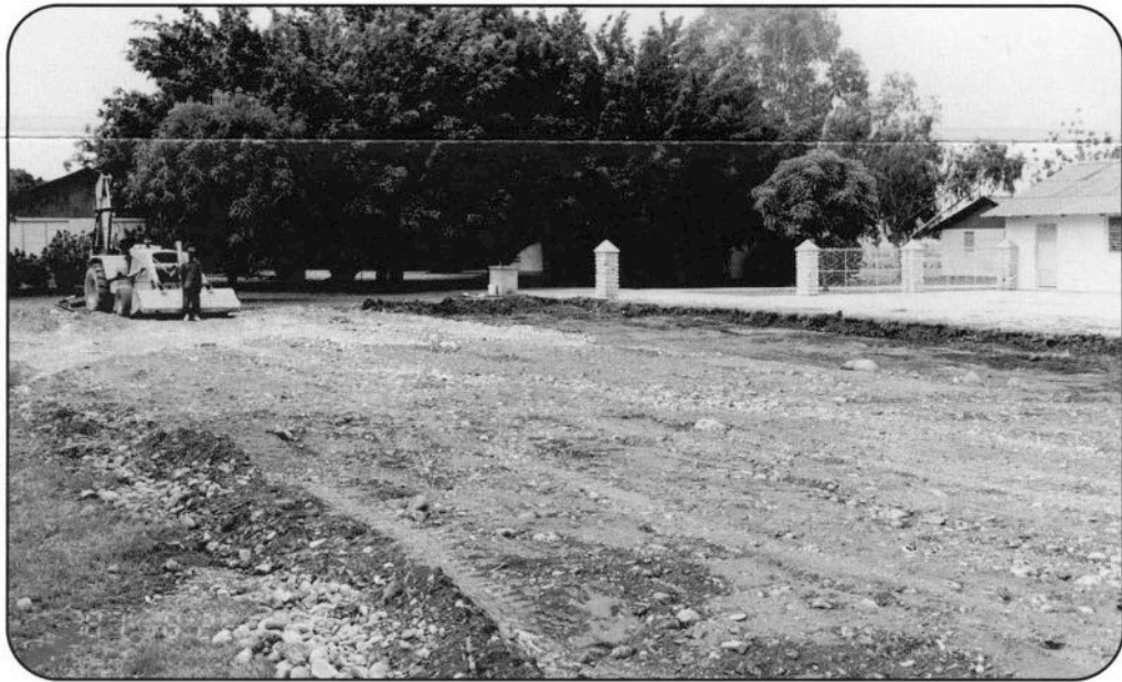
Preparing the site for College expansion.
