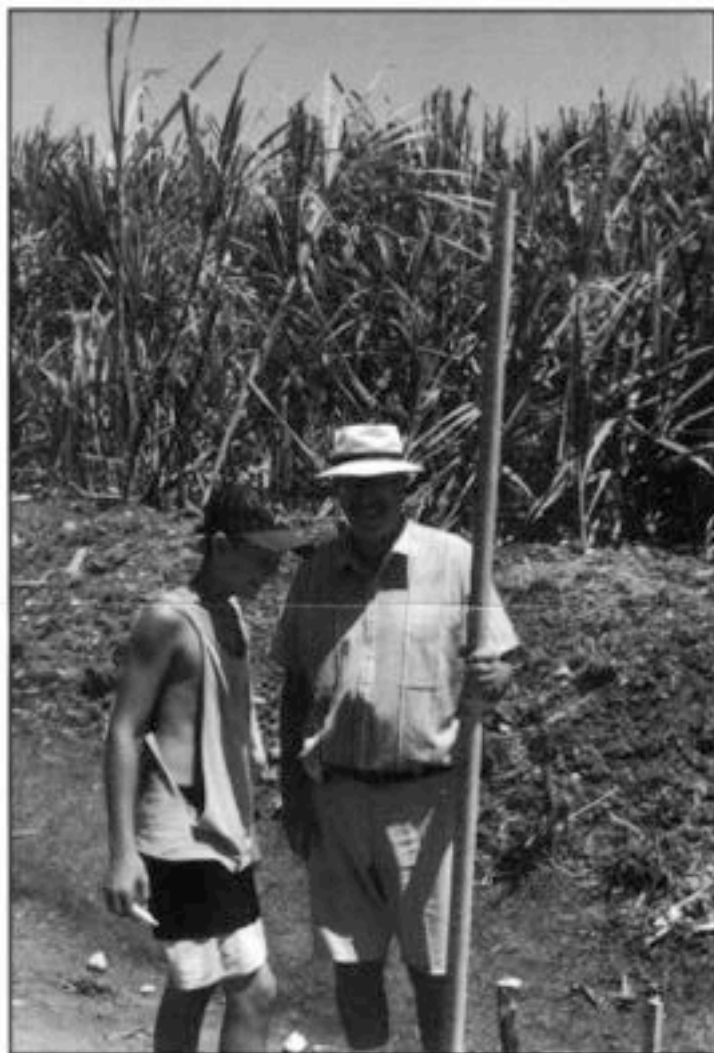
Blair Wagner and Luke Horst enjoyed working together as Blair surveyed during the road construction project.
