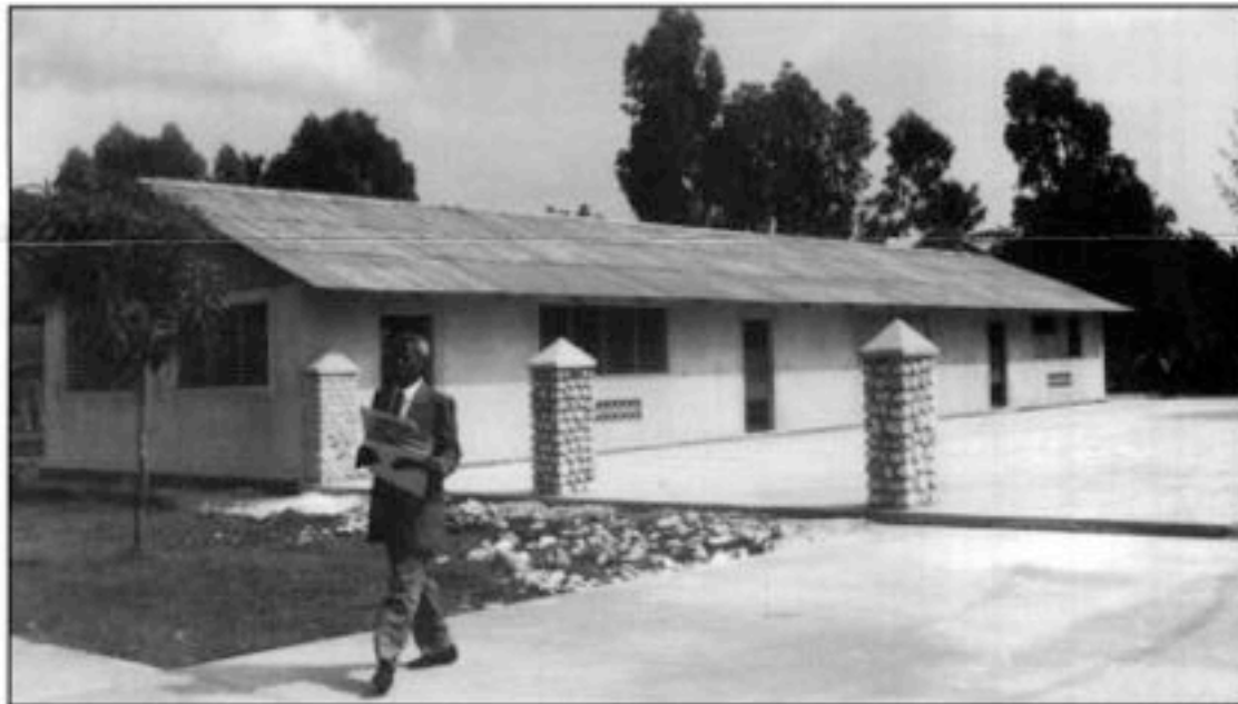
Julian Leandre, director of the high school at New Missions, is walking past the newly completed building that is already being used by our students.
