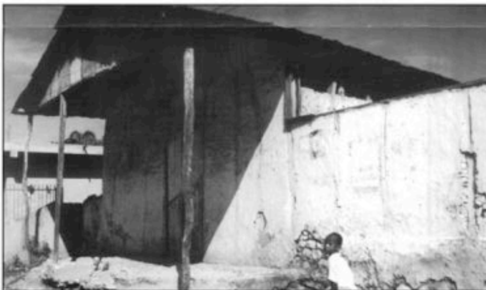
Construction will start this fall for the much needed church building in Leogane. This building will be torn down. This is the front view of the Leogane Church.
