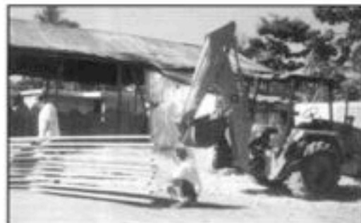
Leogane school construction
