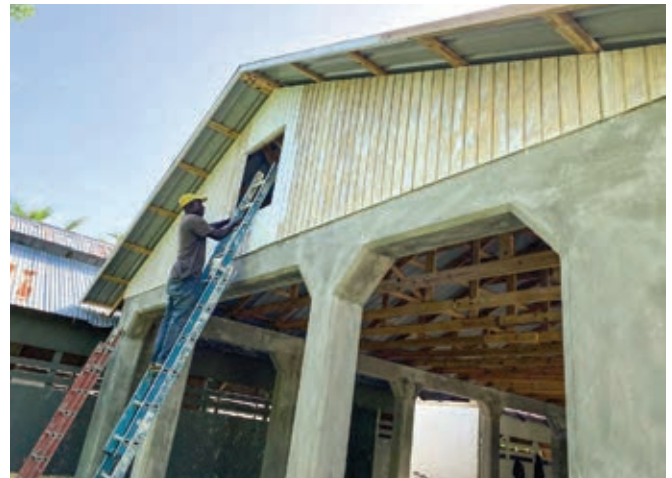
Carpenters from New Missions built the trusses at our mission and then installed the church roof.
